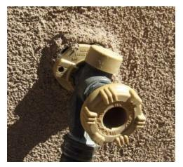
←7- The spigot on the south side of the building is not properly secured to the wall. It should be.
