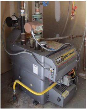
3- The kitchen and living room zone valve was open despite the zone not calling for heat. It should be replaced.
